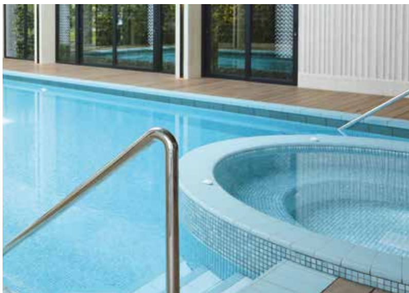
Pool EW 23, Surabaya, Indonesia Architect: Ir. Sonny Njonoriswondo, Surabaya, Indonesia Series: Pool edge system Bamberg, Chroma non-slip. Fresh Photo: George Arif (Spin Production)
