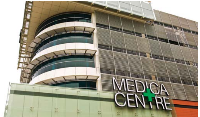
Project: Medica Centre Client: Hansen Yuncken
