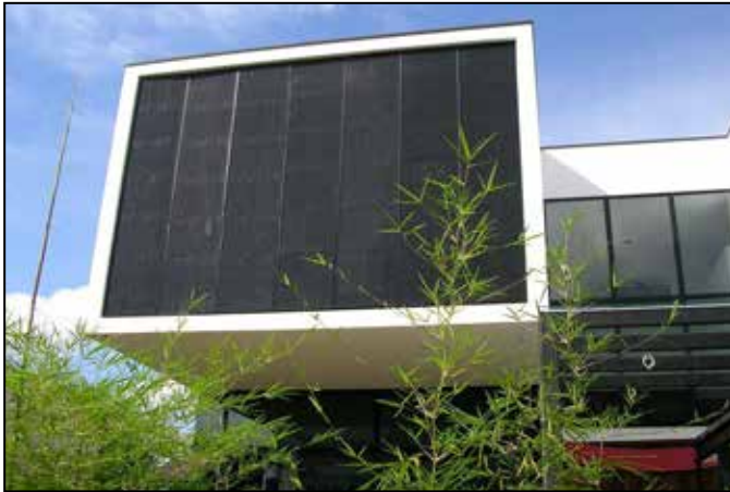
Atlantis Gro-Wall® Facade installed as a shade wall.
