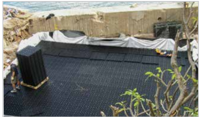
Installation of Atlantis Titan Tank®
