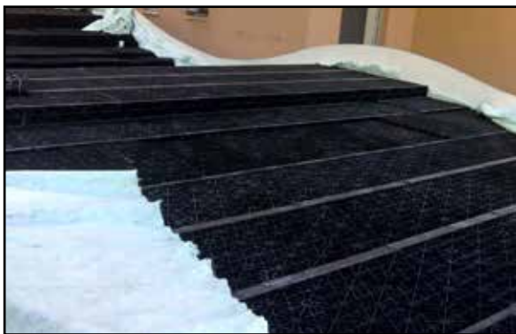
Atlantis Flo-Void® modules used as lightweight structural void fill into landscape planter boxes.
