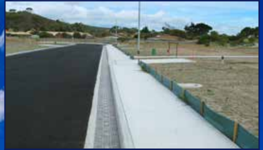
ROAD EDGE INFILTRATION
