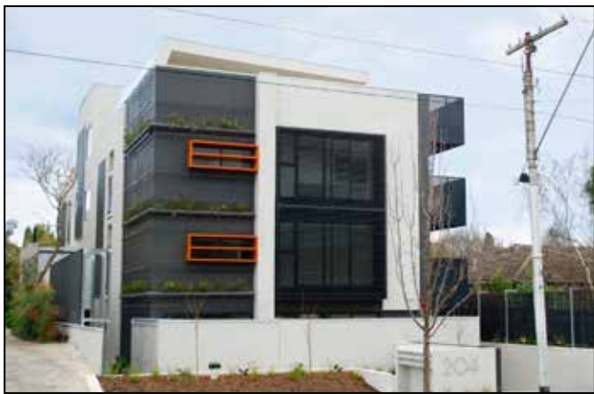
Atlantis 52mm Flo-Cell® installed into apartment building as a screening wall (left) and fence (right).
