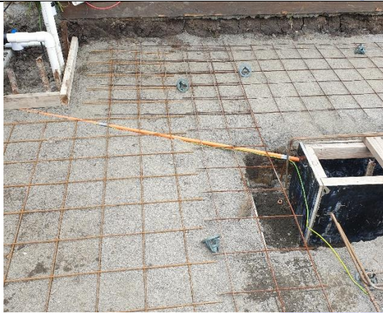
Conduit for power if required
