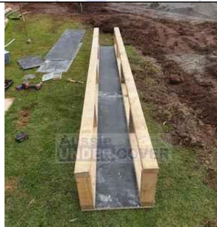
Screw 20mm Form Ply to the four outside edges. Top and bottom left open.
