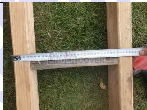
Outside to outside 350mm wide 90 x 45 treated pine. 20mm form ply will be added to each outside edge.
