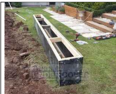
Overall completed formwork = Pit length by 390mm wide x 450/500mm high/deep
