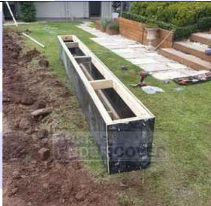
Completed form work 390mm wide x 500mm deep. Length to suit pool & kit
