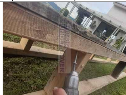
Screws must be accessible once the concrete has been poured so the form work can be removed
