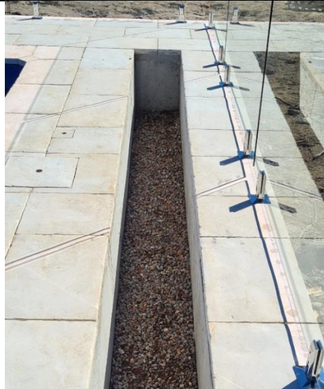
Paving finished flush with pit walls
