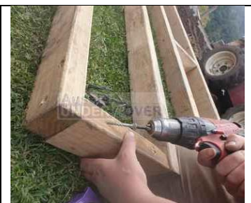
Screws must be accessible once the concrete has been poured so the form work can be removed
