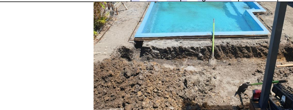
Completed form work 390mm wide x 500mm deep. Length to suit pool & kit
