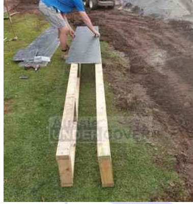
Screw 20mm Form Ply to the four outside edges. Top and bottom left open.
