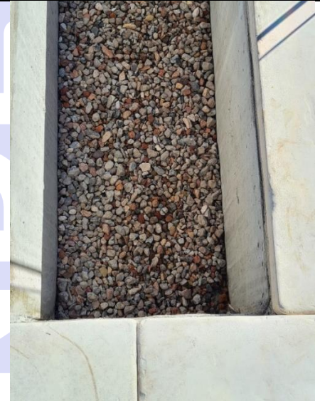
Agi line and Gravel drainage in base
