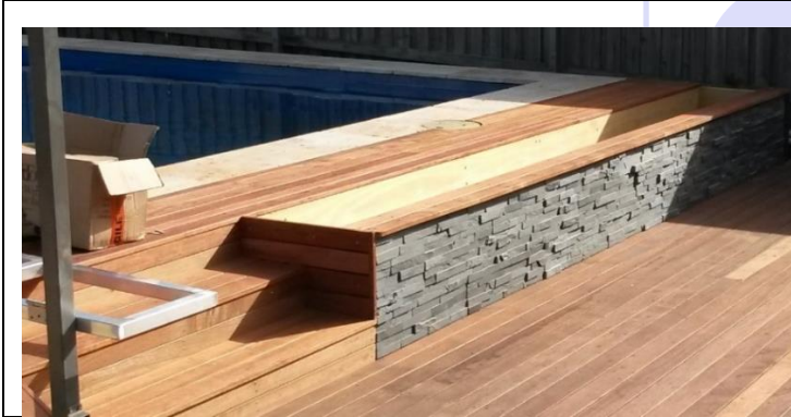
Cavity lining 190 x 35 or 245 x 35 as required
