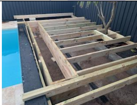
Cavity lining 190 x 35 or 245 x 35 as required
