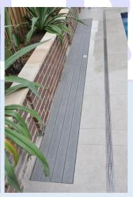
Install chosen lid frame covering ie. decking, composite decking or tiles – install pool cover
