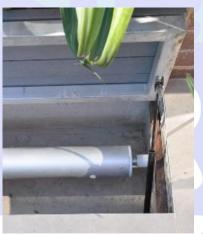
measure, trim (if required) and install lid frame - Install gearbox, end mount and tube assembly
