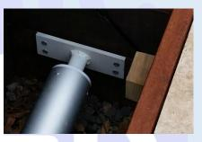
Install framing to create the deck opening required for the kit – mount gearbox, end mount and tube assembly
