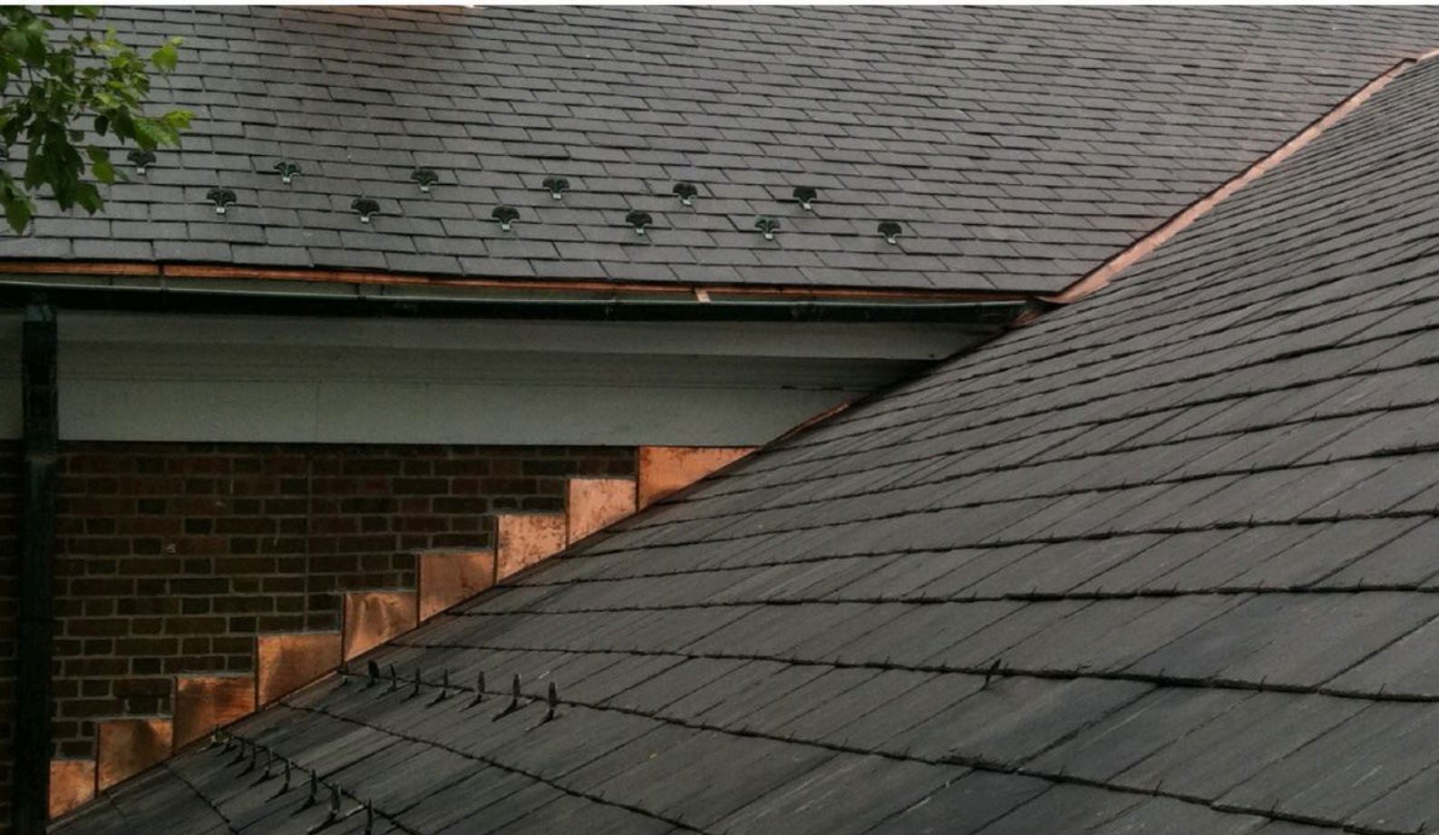
Architectural Slate Roofing
