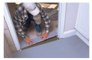
DensShield<sup>®</sup> Tile Backer is lighter and easier to install than leading cement and fibre cement board brands (12.7 mm comparison). DensShield<sup>®</sup> Tile Backer provides excellent dimensional stability and strength so it can be installed parallel or perpendicular to the framing in walls and ceilings.
