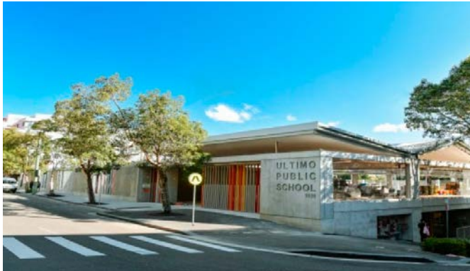
Project: Ultimo Public School Client: Hindmarsh Constructions
