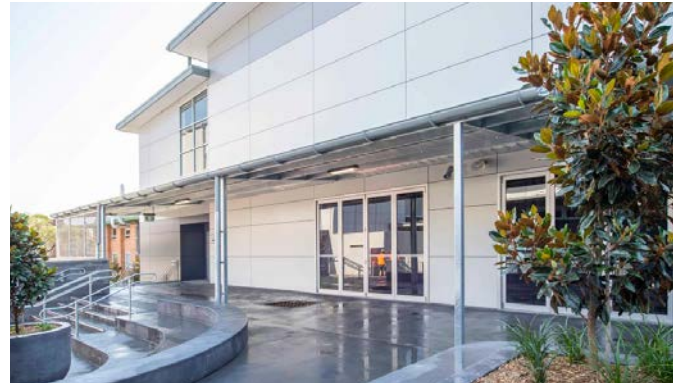
Project: Hunter School of Performing Arts Client: Richard Crookes Constructions
