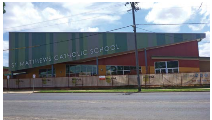
Project: St Matthews Catholic School Client: Farindon Constructions
