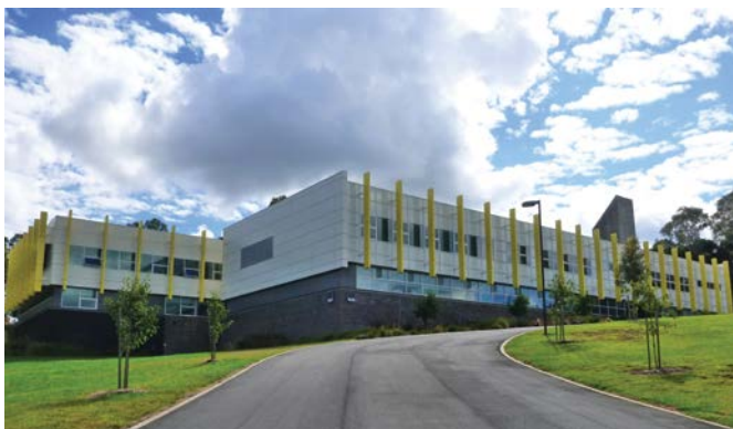
Project: CSU Orange Client: Zauner Constructions
