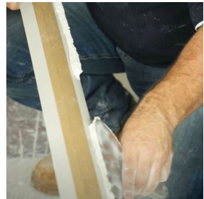
3. Apply Cornice adhesive
