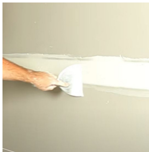
First Coat - Bedding compound
