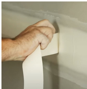
First Coat - Taping
