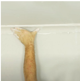
4. Position the cornice
