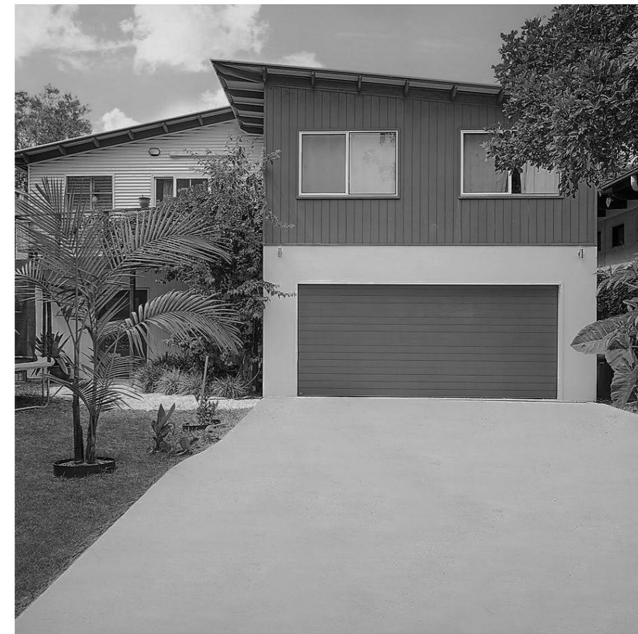
EXISTING STREET FACADE
