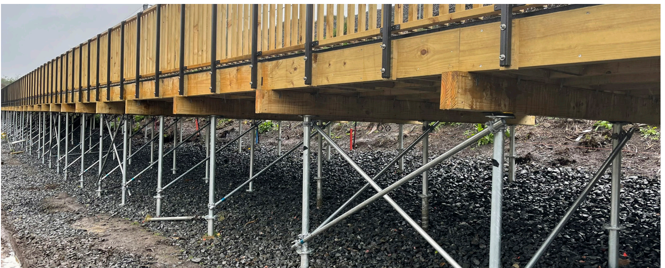
SGC EL is well suited where floods are possible, or where damage or disturbing of the ground is restricted.
