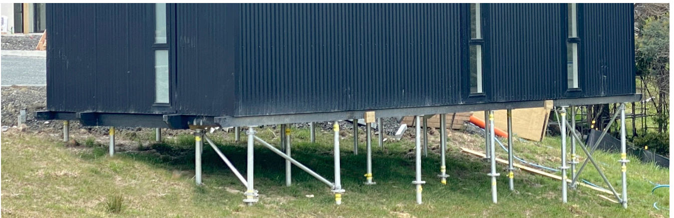
For house foundations, transportable buildings and decks in sloped areas, or poor soil where it would be very expensive to dig out and use concrete slabs etc.
