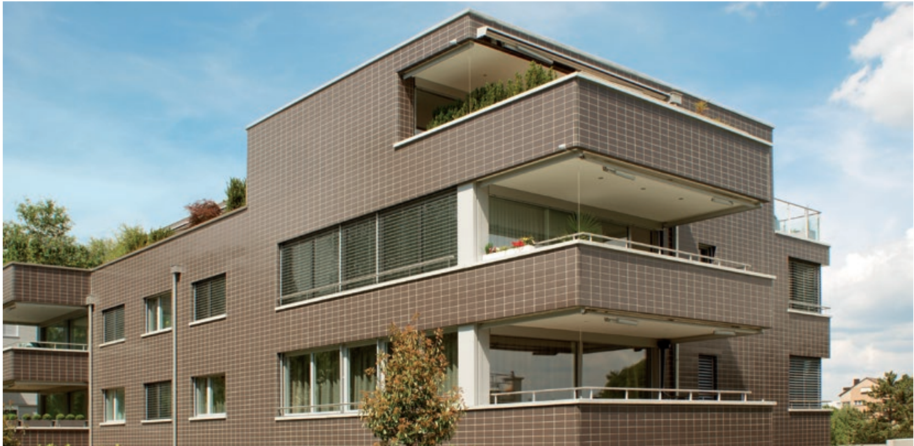
Apartment building, Kilchberg, Switzerland Architect: Horizon Architektur + Bau AG, Zurich, Switzerland Products: Chroma II, special colour
