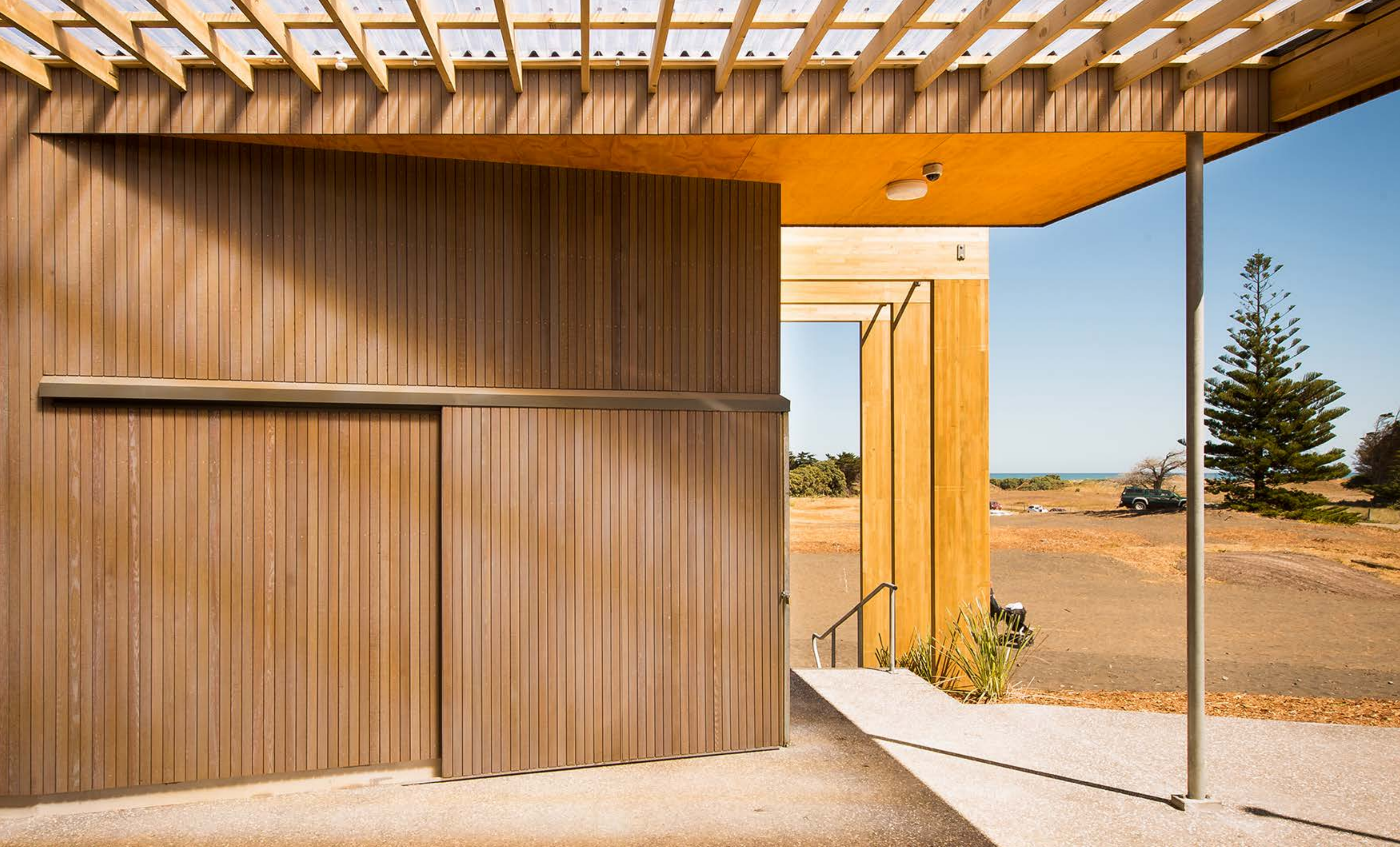
VERTICAL SHIPLAP CEDAR WEATHERBOARDS Muriwai Surf Club
