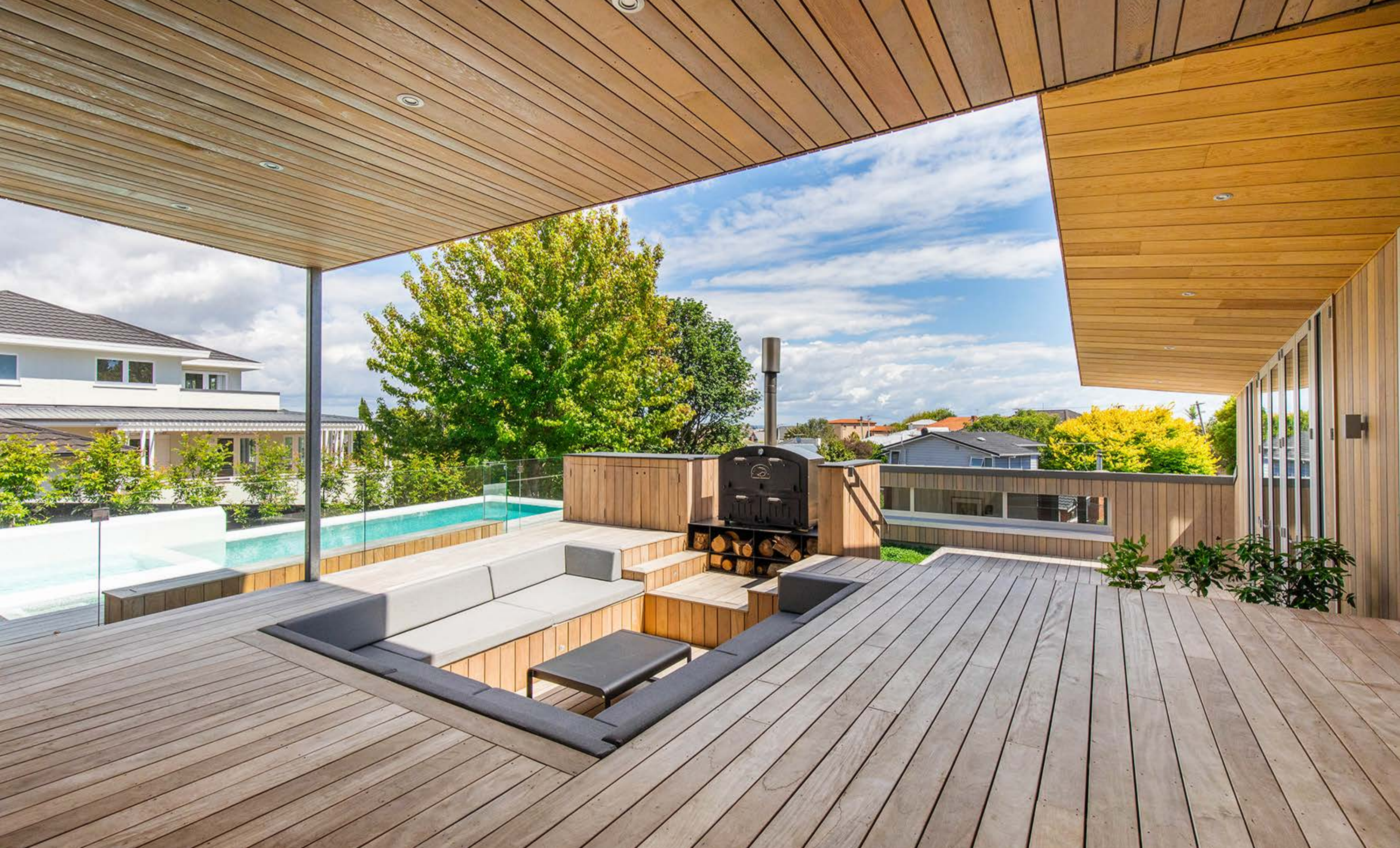
RANDOM WIDTH CEDAR WEATHERBOARDS, VITEX DECKING Private Residence
