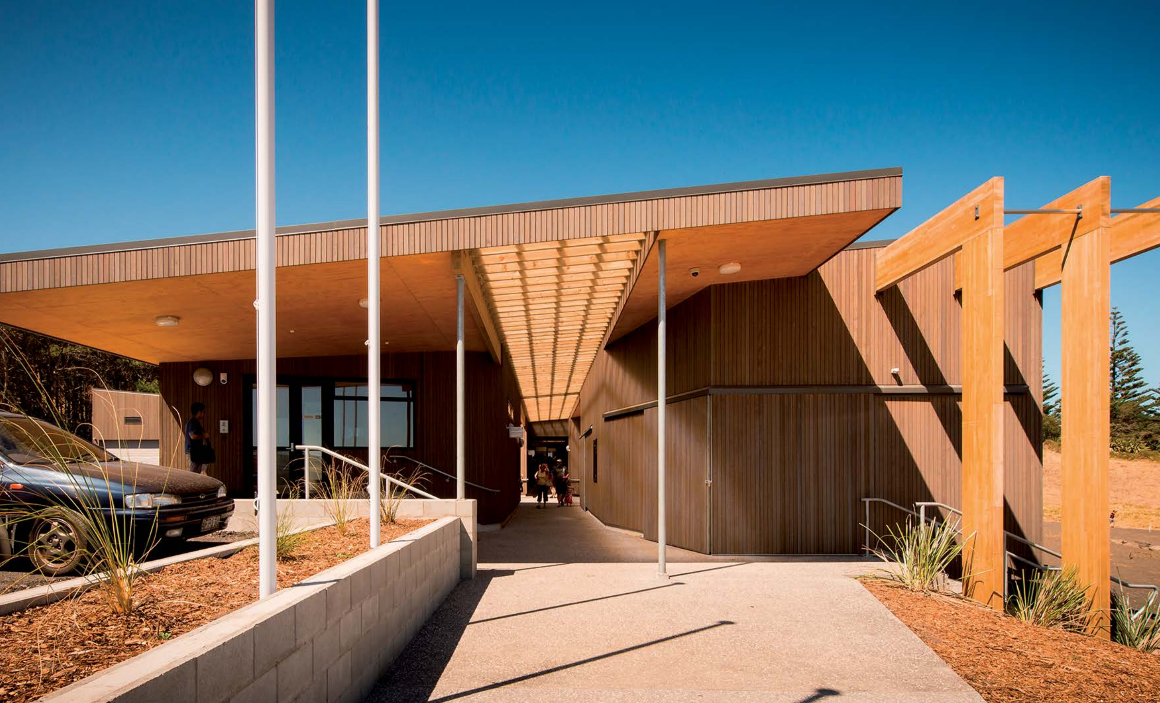
VERTICAL SHIPLAP CEDAR WEATHERBOARDS Muriwai Surf Club
