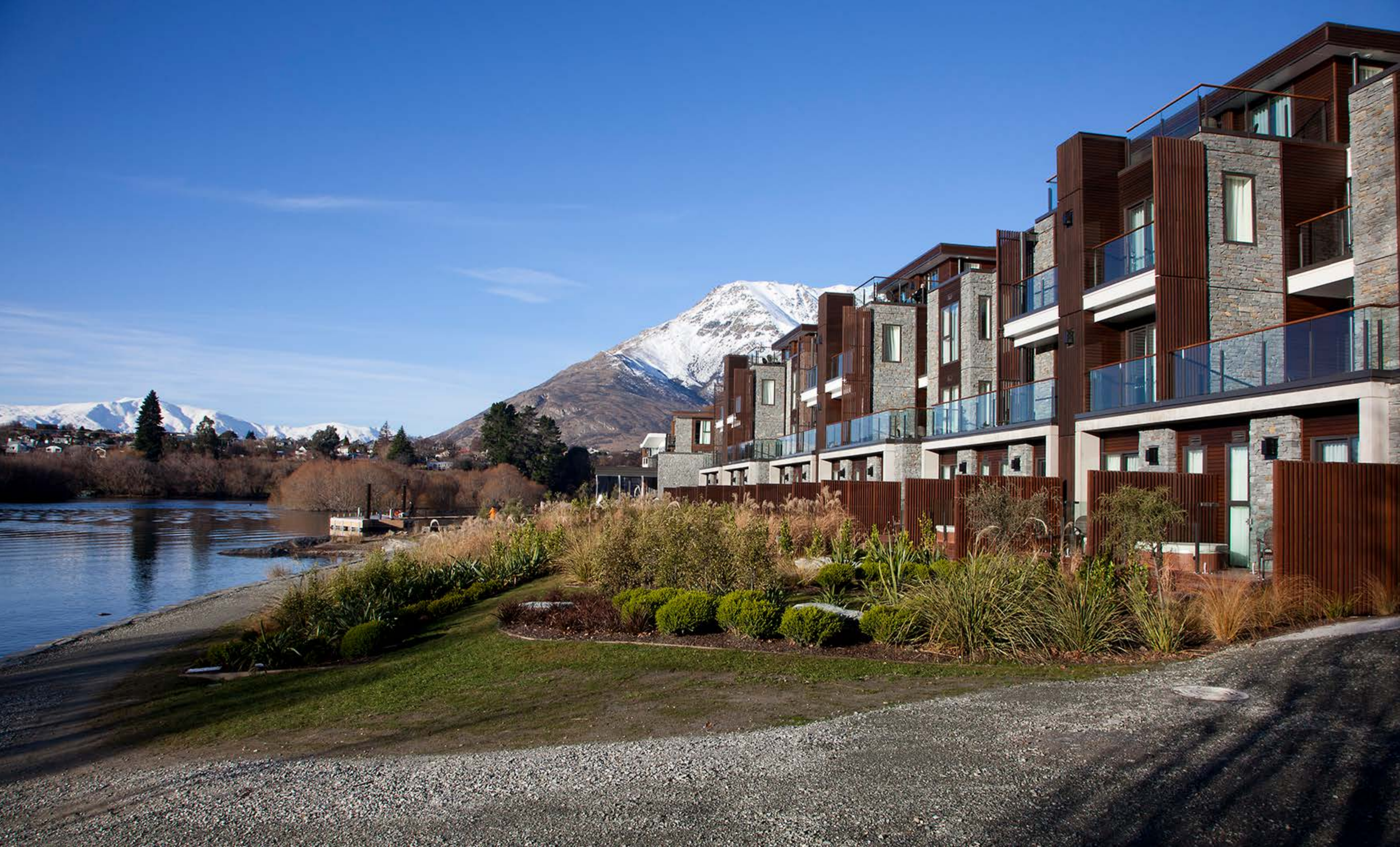
RUSTICATED CEDAR WEATHERBOARDS, VITEX DECKING Hilton Resort & Spa, Queenstown
