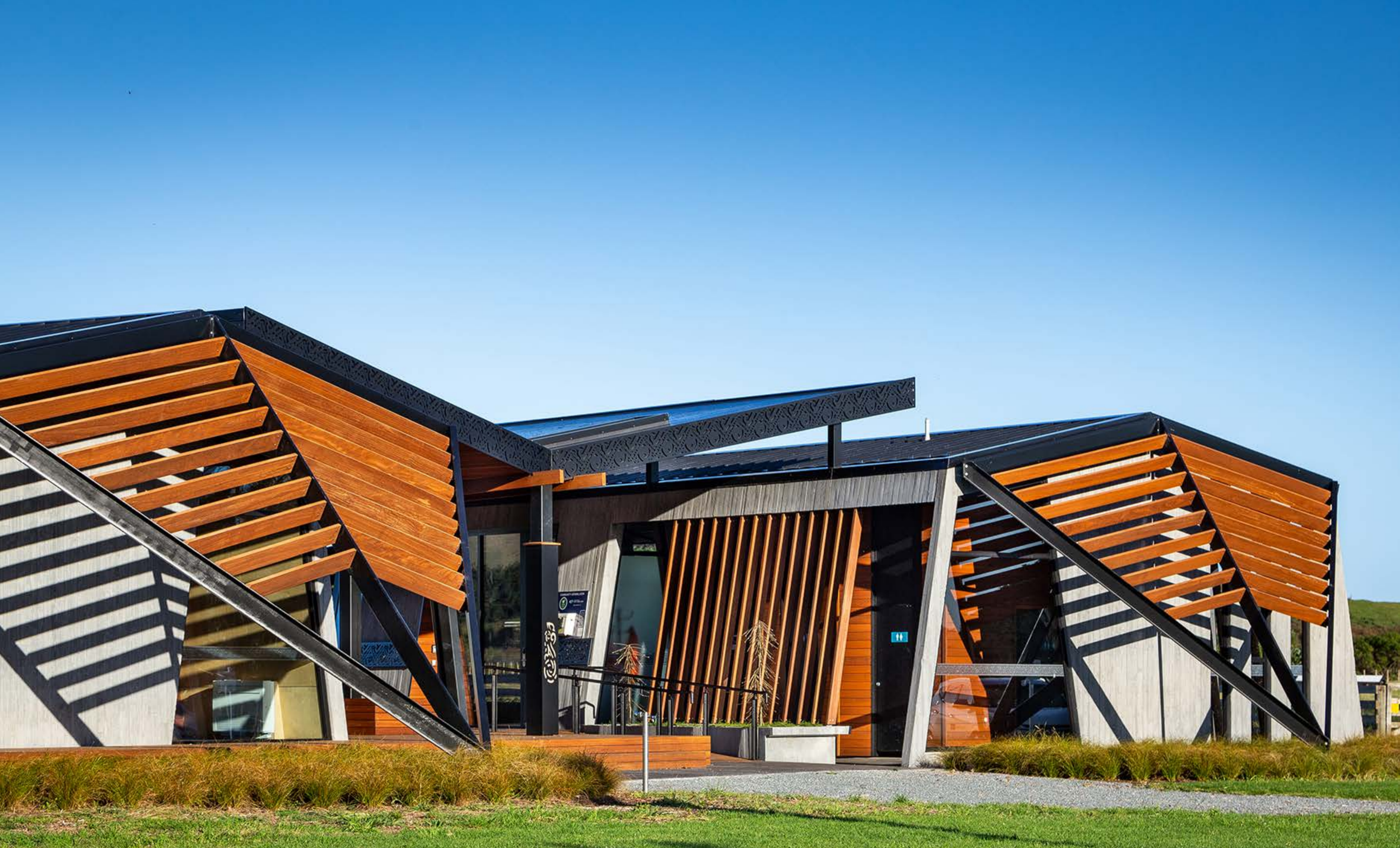
IROKO DECKS & FINIS Ramaroa Heritage Centre, Kapiti Coast
