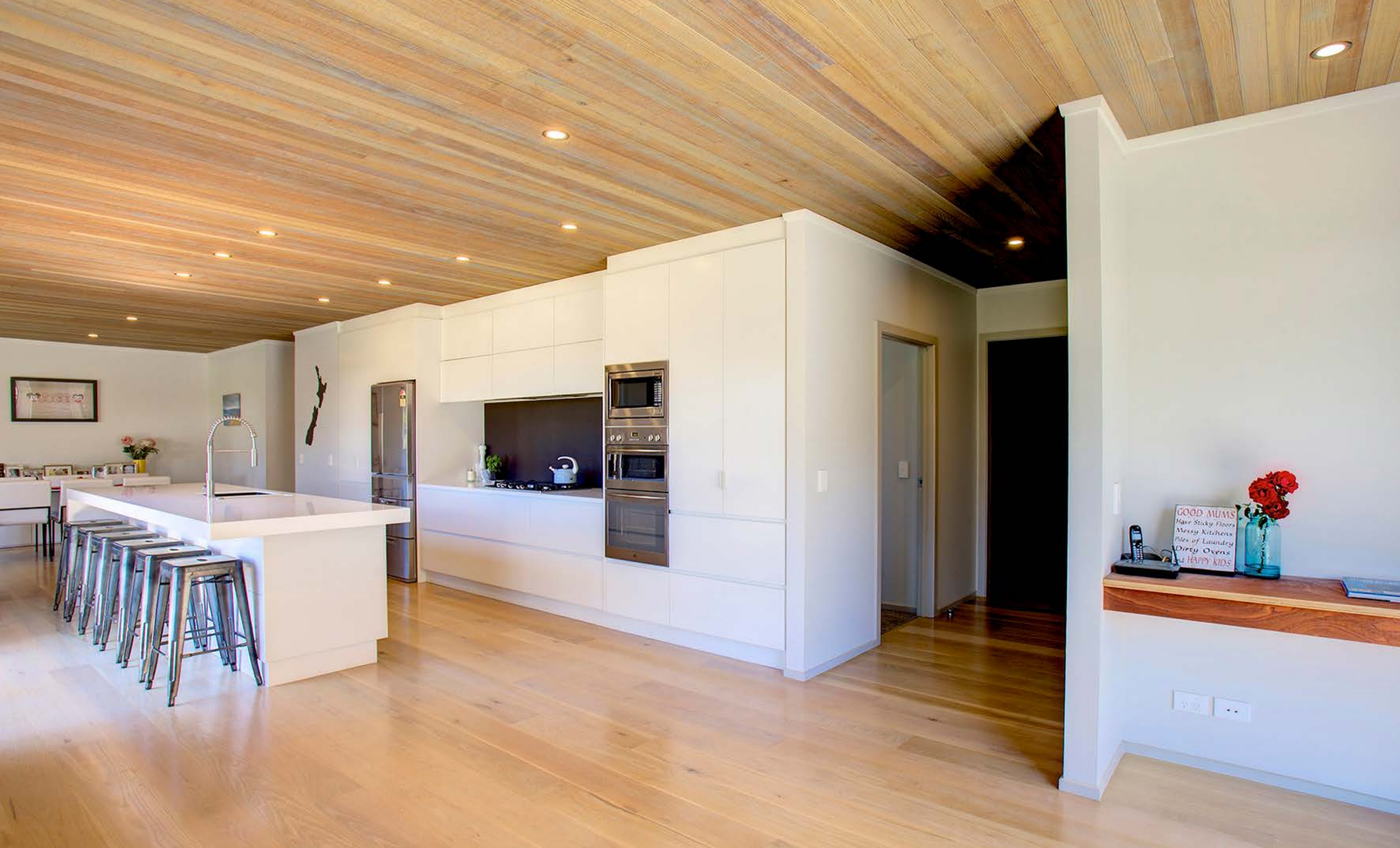
CEDAR PANELLING, SOLID AMERICAN WHITE OAK FLOORING Private Residence
