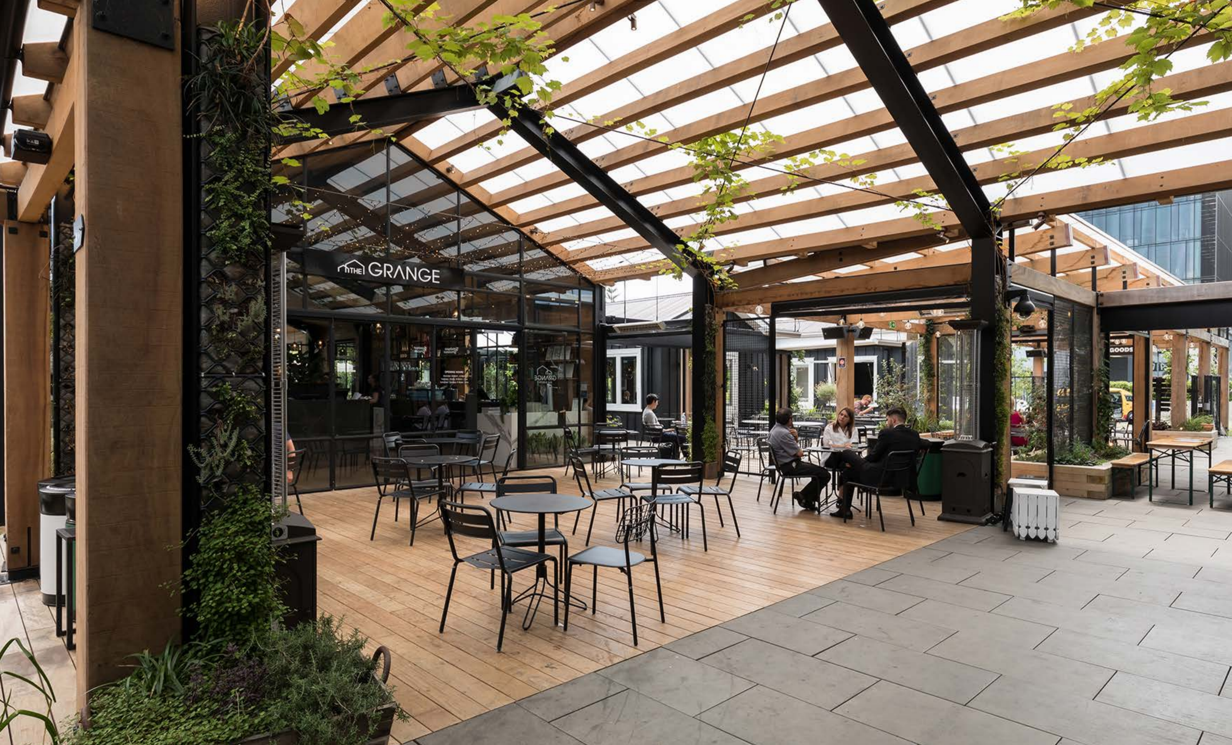
CUMARU BEAMS, VITEX DECKING Goodside, Smales Farm, Takapuna
