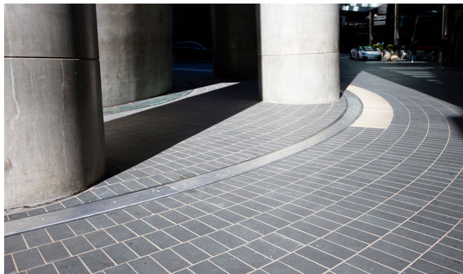
Technically challenging radial paving
