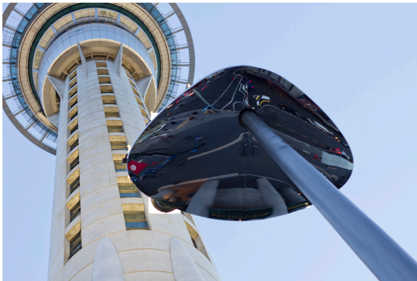
A bespoke 17m high flood light gantry enabled the reduction in structures at the base of the tower - the design including a reflective dish is conscious to contribute to the space without attempting to compete with the tower.
