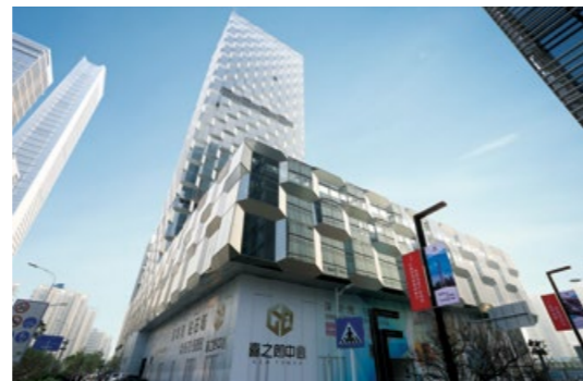
Strong Group Headquarter Building
