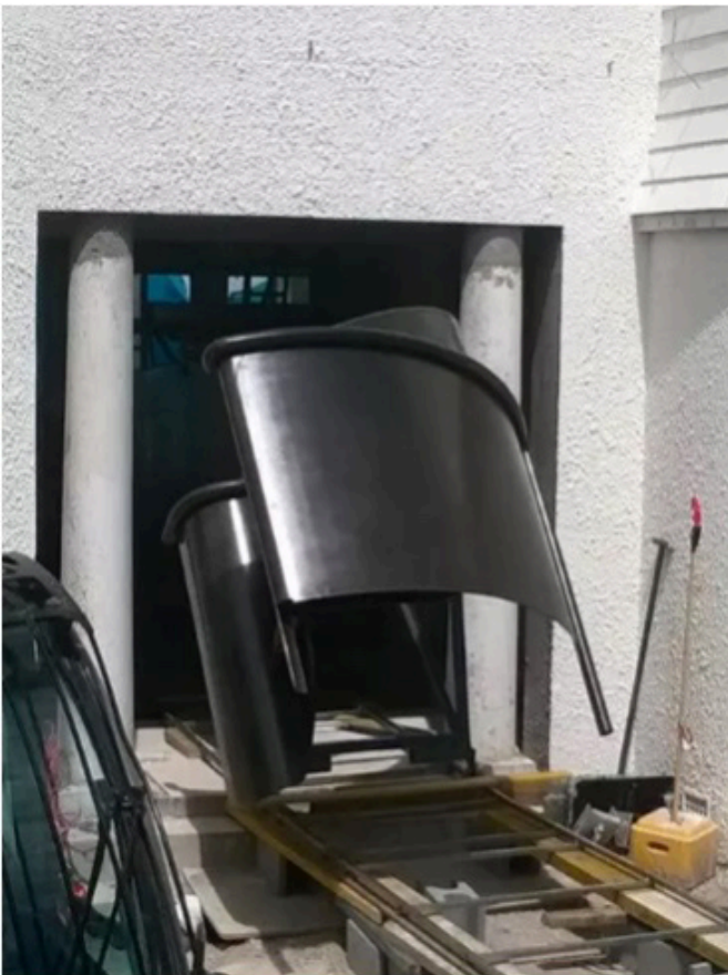
The in-situ shots above show the complexity of the install, which involved the creation of a rail cart system to access the site via a ramp, with the stair sections guided into place, squeezed through the front entrance and chain lifted into the stair void and massaged into position.
