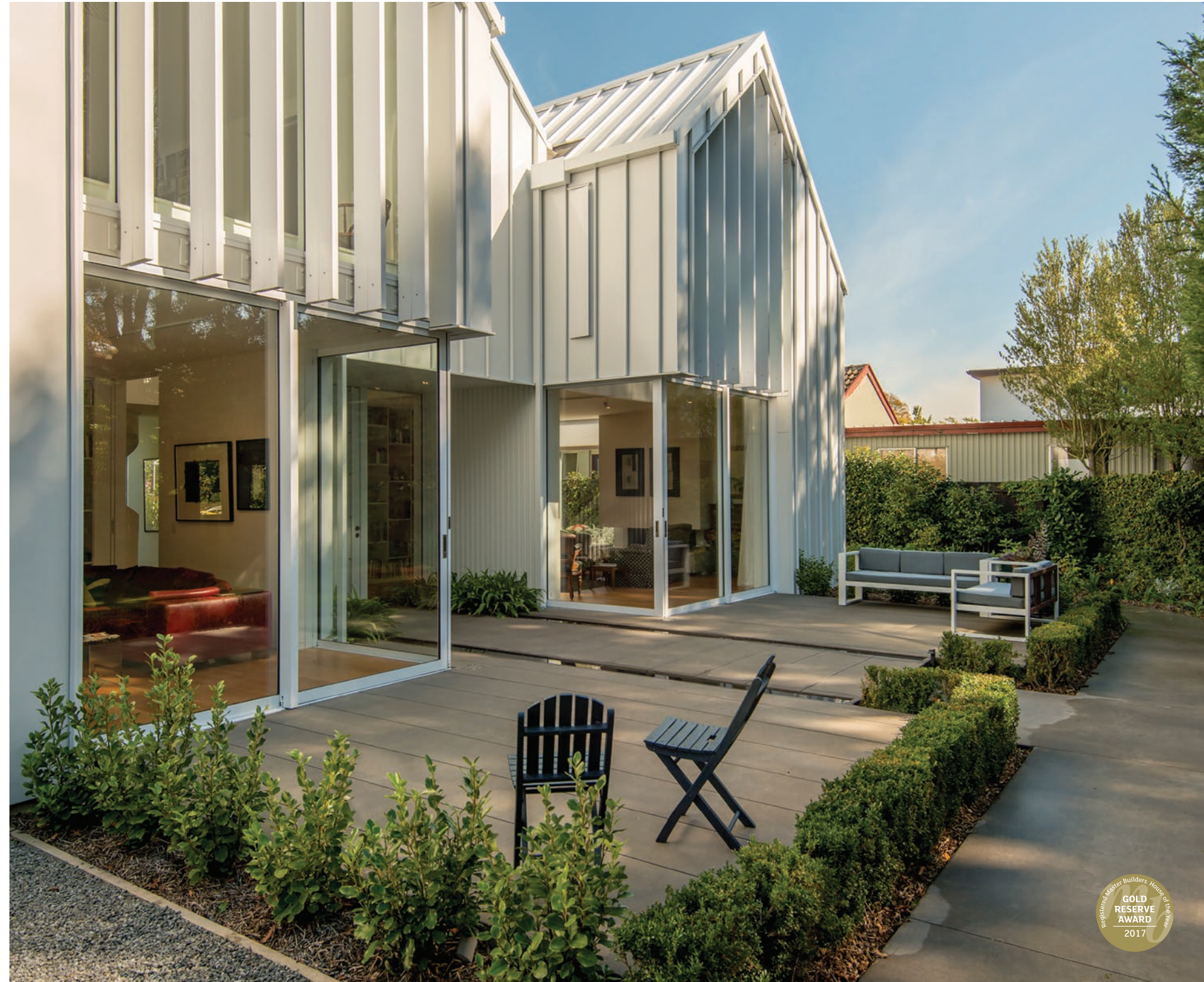
C Fendalton House North elevation showing the metal cladding, aluminium windows and form in its entirety. Intricate detailing was required throughout the house with this elevation highlighting its complexities.
