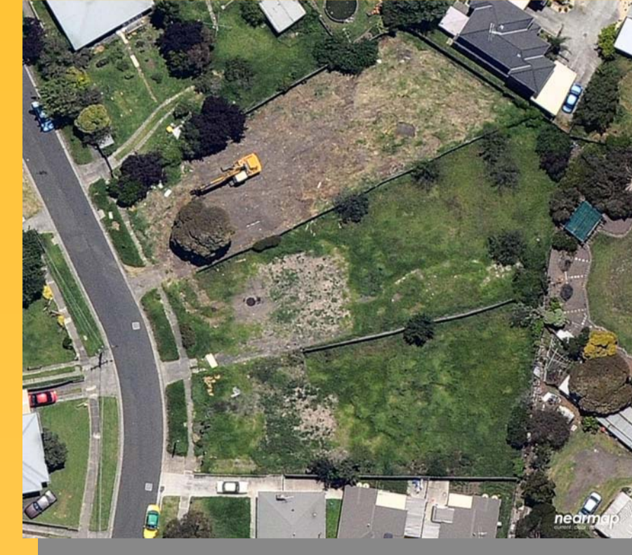
Melbourne Basaltic Tertiary clay in Braybrook; Victoria
