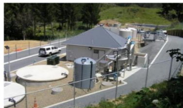
Kawakawa Bay WWTP, Watercare Services Ltd
