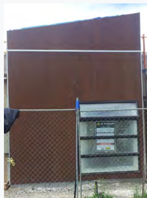
0 MONTHS: Recently built, this shows the beginning colour of Weathertex Natural boards.
