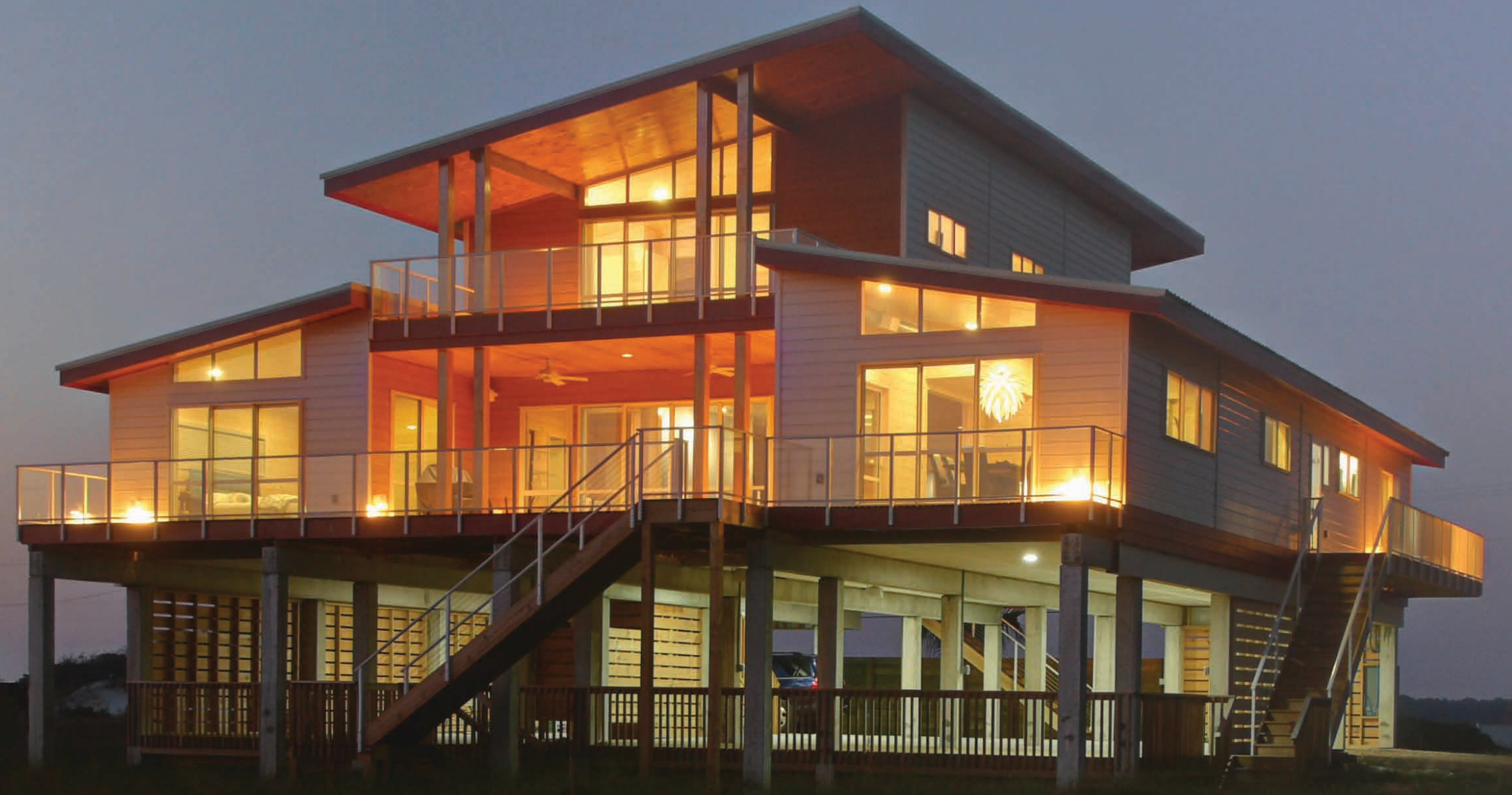
This Lockwood home in Alligator Point, Florida, withstood 230km/hr winds and huge seas as the Category 4 Hurricane Michael hit the coast of the USA late 2018. It was one of the few homes in the neighbourhood to survive unscathed.
