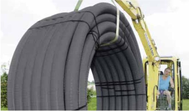
Fig. 40 Lifting with a digger
