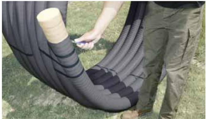
Fig. 44 Cutting the coil straps
