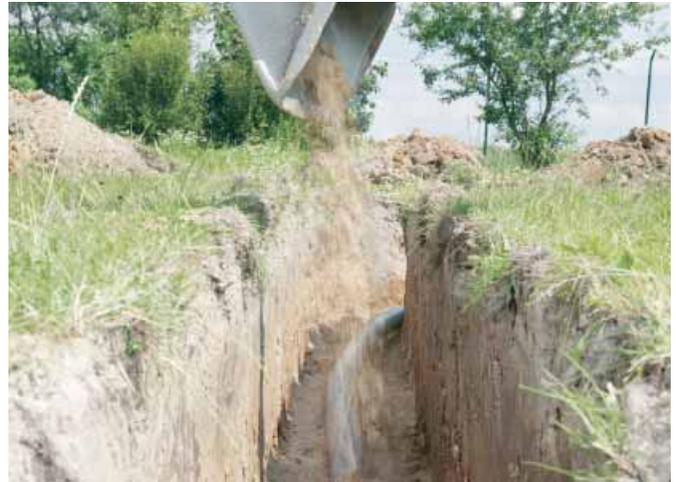
Fig. 49 Backfilling trenches with sand
