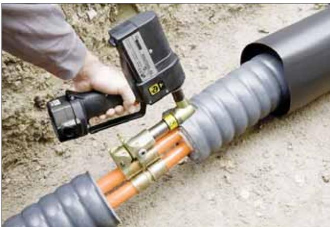
Fig. 2 RAUVITHERM compression sleeve joint
