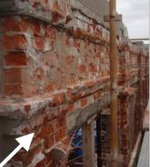
The majestic building was restored by chipping loose material away from the structure and then rebuilding it.
