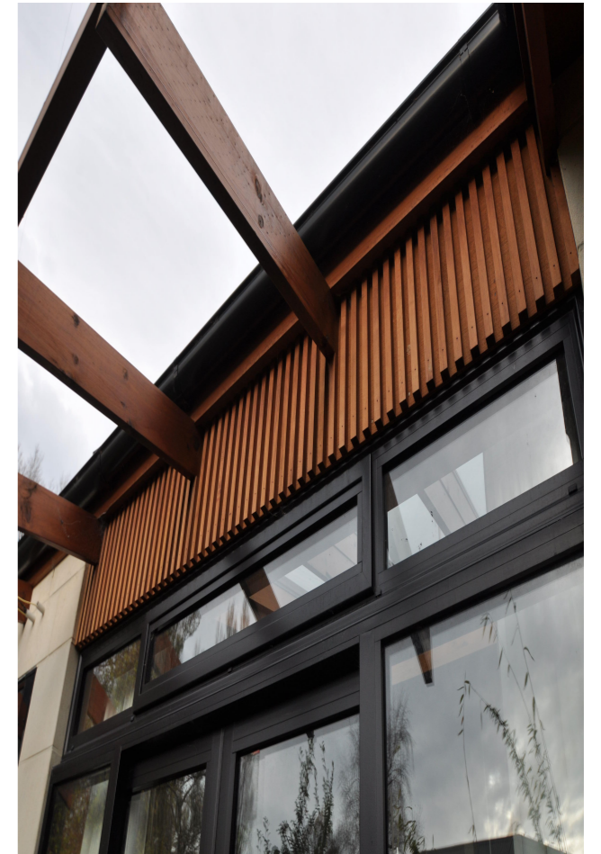
Eaves are cut away at the conservatory & solar panels
