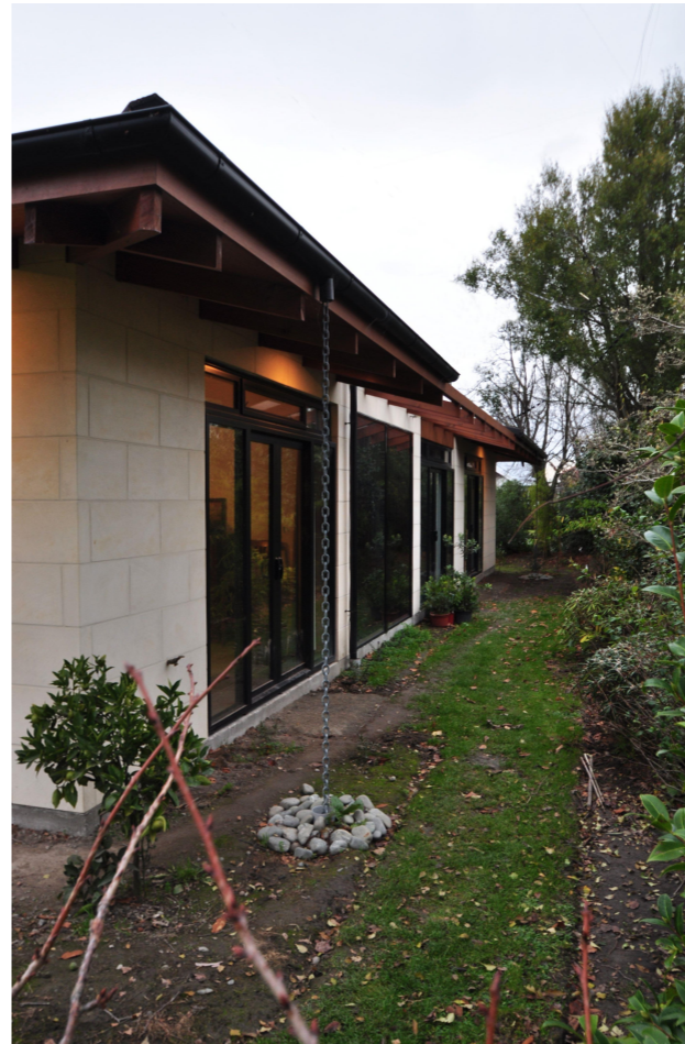
Wall mounted solar panel look like windows
